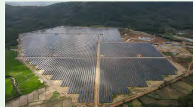
Mega solar power plant in Binh Dinh Province
