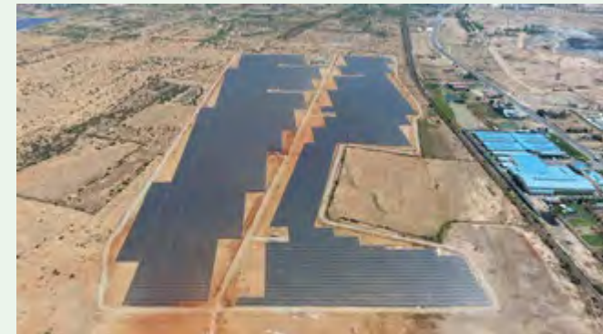
Mega solar power plant in Ninh Thuan Province
