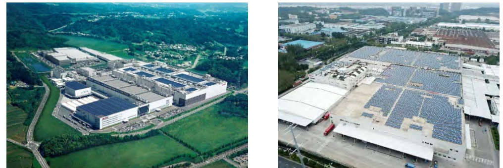
Solar power systems installed on the roofs of Sharp production bases (left: Kameyama Plant; right: NSEC in China)
